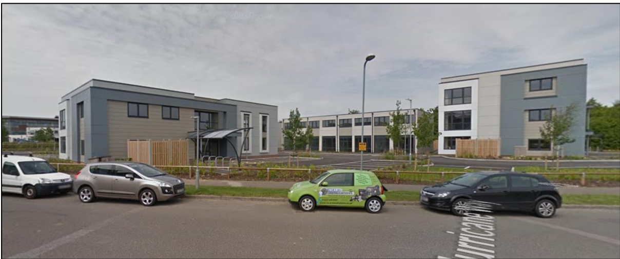
(Left to right) Blocks C, B, and A as seen from junction of Hurricane Way and Defiant Close
